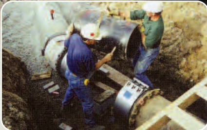
▲ Repair work for pipes replaced underground
