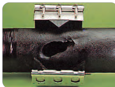
▲REPAIRING THE PIPES
