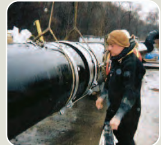
▲ UK: district heating work
