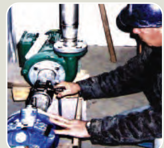
▲ Repair work for high-pressure pump and water supply pipe
