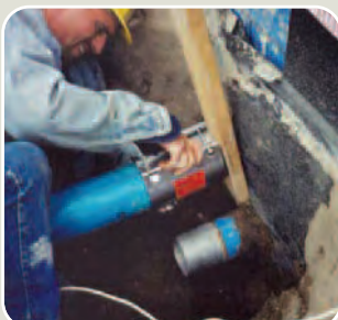
▲ U.S.: sewerage repair work
